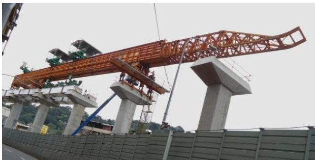
發進吊裝工作車 (LAUNCHING GANTRY)
