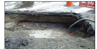
Fig. 6 Excavation of Xinbeitou \phi 300 mm DIP Leak Point
