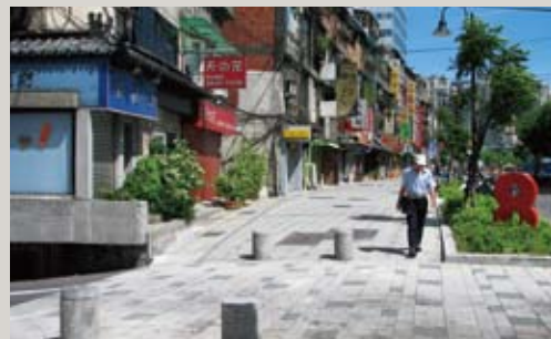
After Renovation - Westside, Xinsheng North Road (Nanjing East Road to 119 Lane, Linsen North Road).
