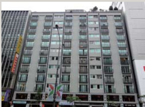
Lingyun Building, after Renovation.
