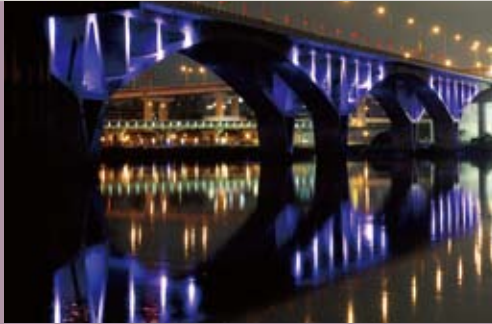
Lighting Design at Wanban Bridge.
