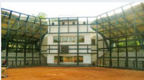
Youth Park Renovation Project.
