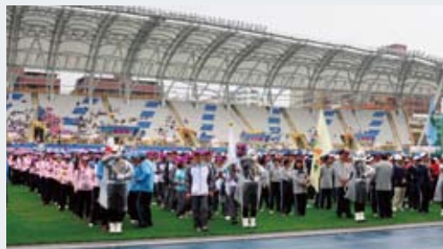
Taipei Track and Field Stadium.
