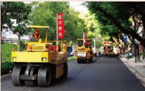
Construction for the road smoothing project (section 7 on Zhongshan North Road).
