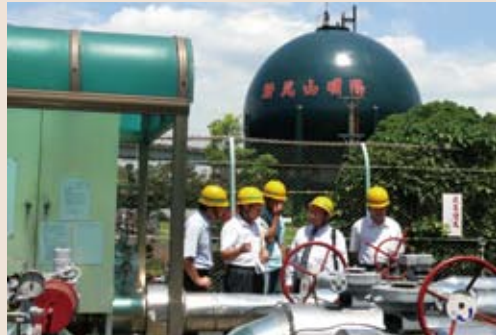
Inspecting gas tank facility maintenance at gas companies.
