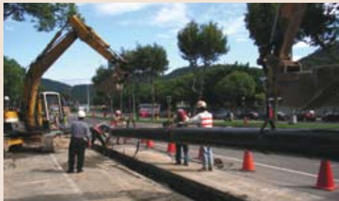
Pipeline network improvement.
