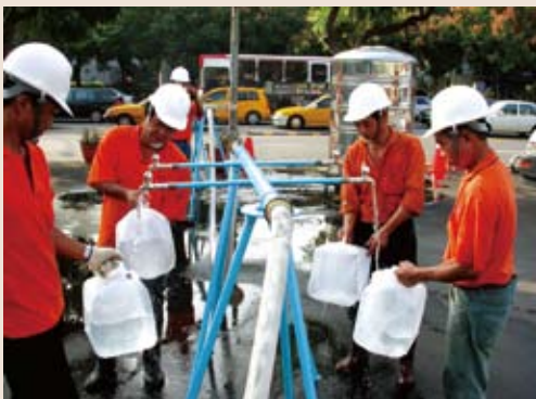
Emergency water access unit.
