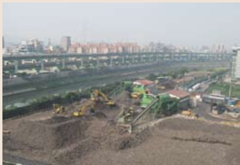
Sifting is conducted at the construction site designated for removing the Neihu Garbage Mountain.
