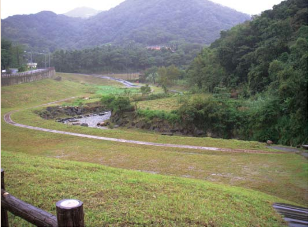
Flood-routing sand basin on Dahu's Shangzhuang Street.
