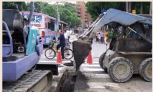
On-site construction where bottom ash is processed for reuse.
