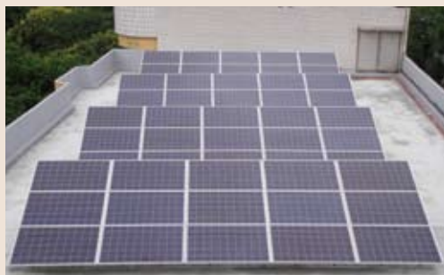
Wanfu Elementary School receives subsidies to design and install a photovoltaic power generation system.
